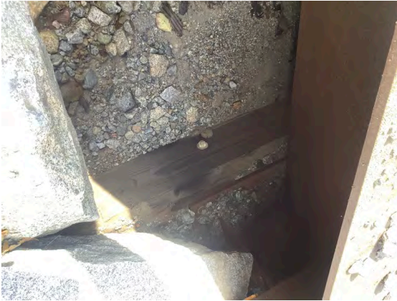
Left Bank Abutment when facing downstream
